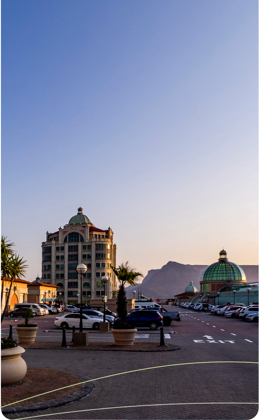
Canal Walk, Western Cape, South Africa
